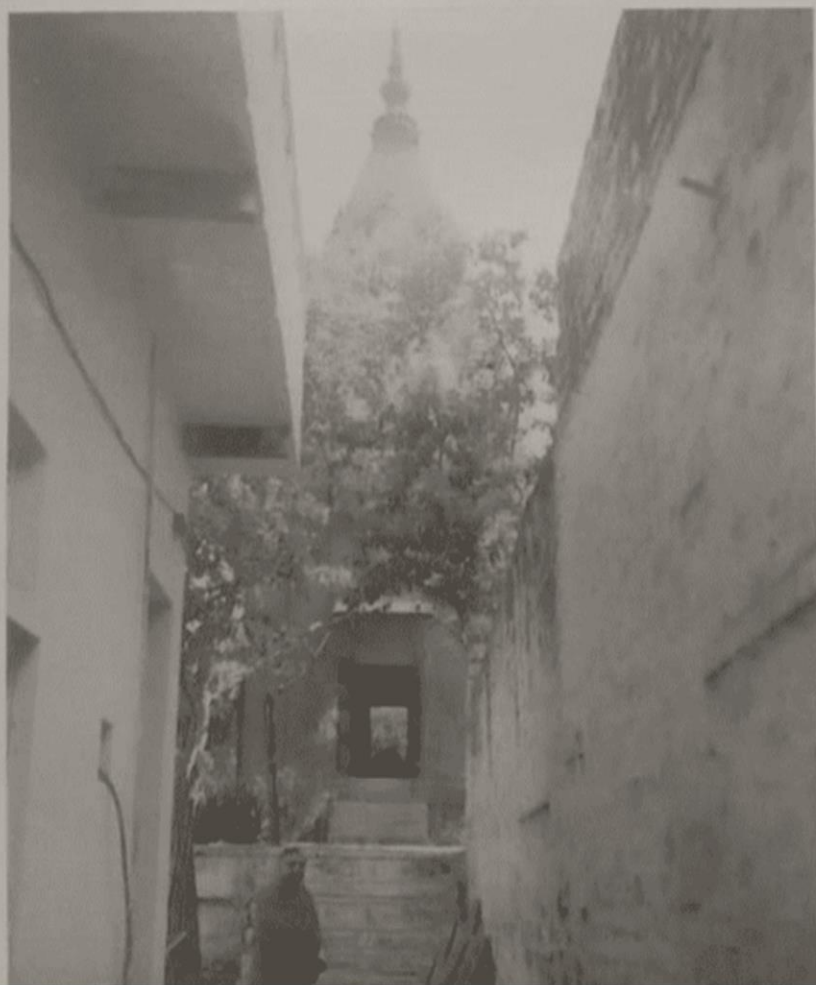
III. 4. ( below ) Kṛtīvāśeśvara temple, as today.
